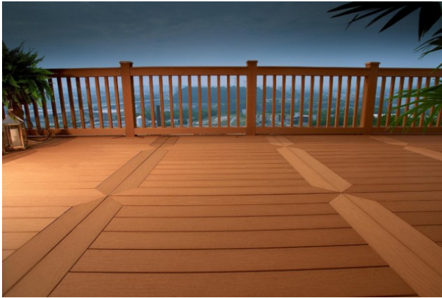
Photo of installed decking
